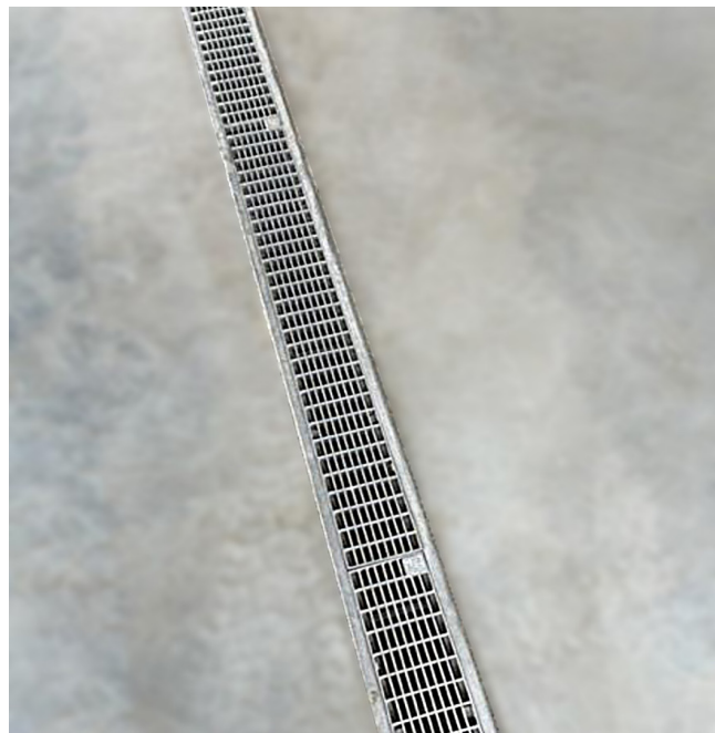
Brown- Forman Distillery Project - Kentucky
