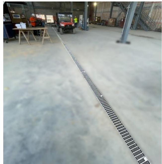
Brown- Forman Distillery Project - Kentucky
