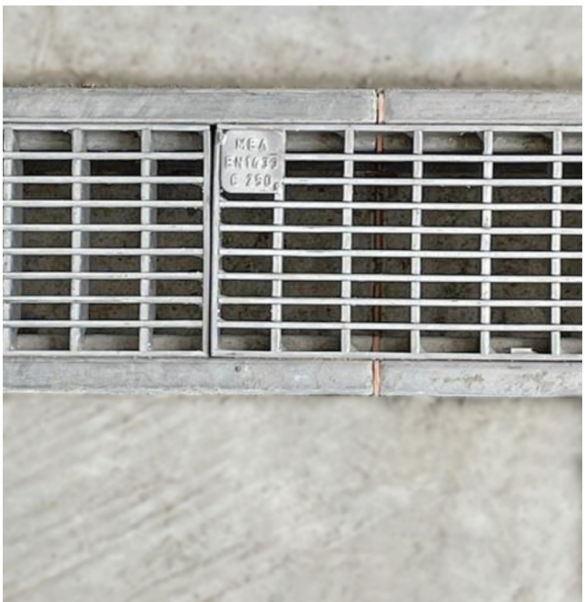
Brown- Forman Distillery Project - Kentucky
