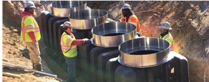
**Installation Overview:** MIFAB provided two SuperMax HDPE Oil Interceptors with 750 gallons of liquid holding capacity and 36" diameter custom lids for a massive public transit project called Purple Line in Landover, MD.
