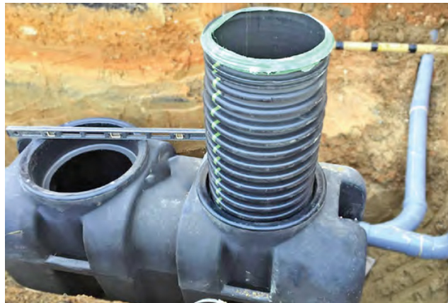
Bayer's Plumbing chose MIFAB's cut-to-fit risers for a client's grease interceptors because they make installation cost-effective and simple.
