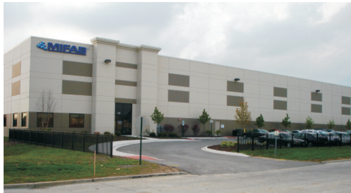
MIFAB's factory in Chicago, Illinois
