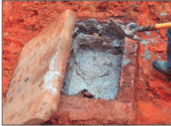
Corroded Concrete Interceptor Typical life expectancy is 10 years.
