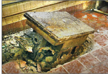
Rusted Steel Grease Interceptor Typical life expectancy is 5 years.
