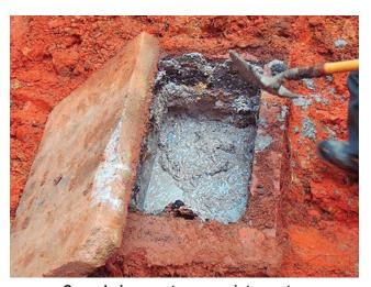
Corroded concrete grease interceptor
