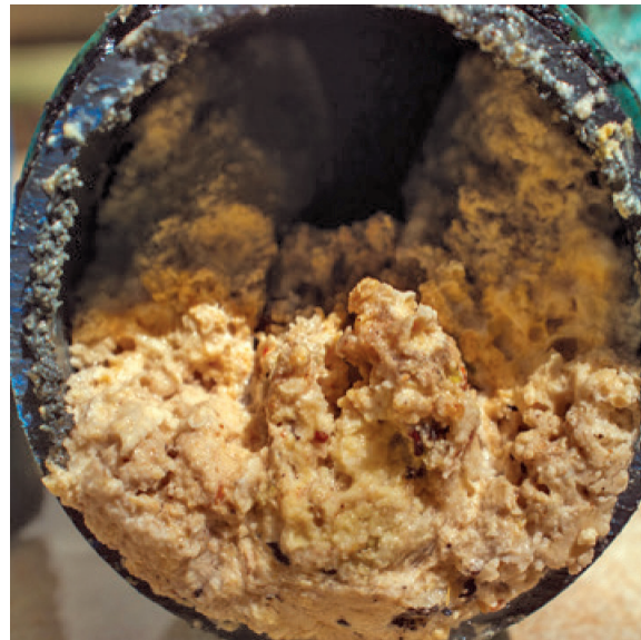
Pipe clogged with grease
