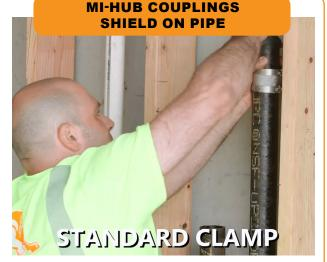
Fastest installation in the market. Fits easy and effortlessly onto pipe. No need to roll gasket. No need to waste time with a loose shield. Fast !
