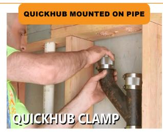
With QuickHub, the contractor simply pushes the coupling onto the pipe. There is no need to remove the gasket first and roll it over the pipe. QuickHub is tested and certified to ASTM C-1277, CISP 310-2010, CSA B602-2010 and is listed with I.A.P.M.O. Available in sizes from 1 1/2" to 12".
