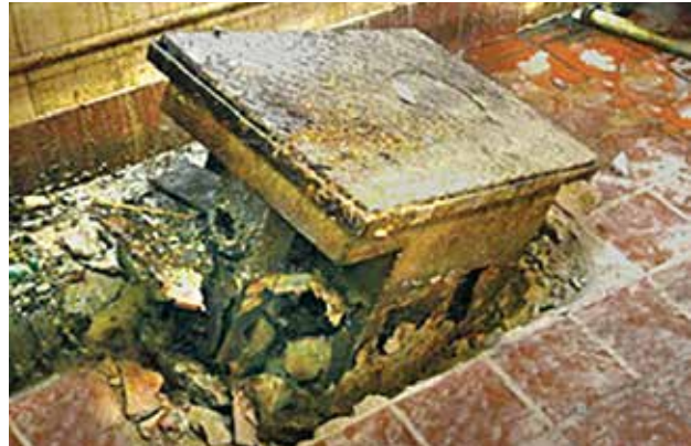
Rusted steel grease interceptor
