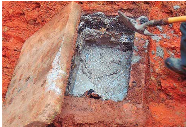
Corroded concrete grease interceptor
