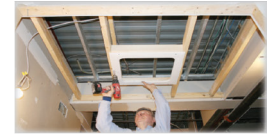
2. Mount Seamless™ surround with drywall screws.
