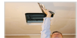
5. Tape and apply drywall compound.
