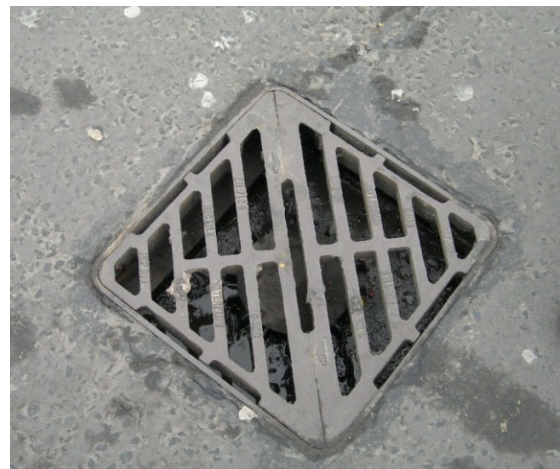
Car Park Drain
