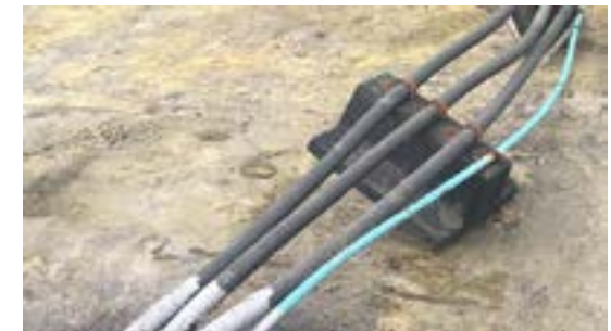
THE COMPETITION Flimsy rooftop supports. These are dangerous.
